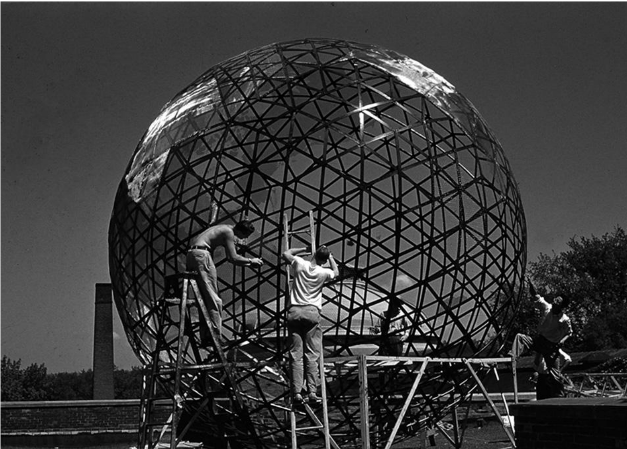
↑ Geoscope (‘Mini-Earth’) prototype under construction at Cornell University, 1952. Courtesy of Estate of R. Buckminster Fuller and Stanford University Libraries, Special Collections, R. Buckminster Fuller Collection.
